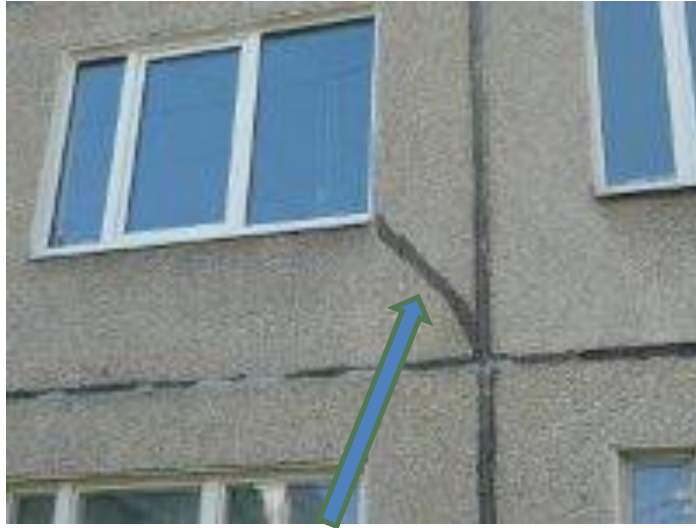
Crushed panel joints
