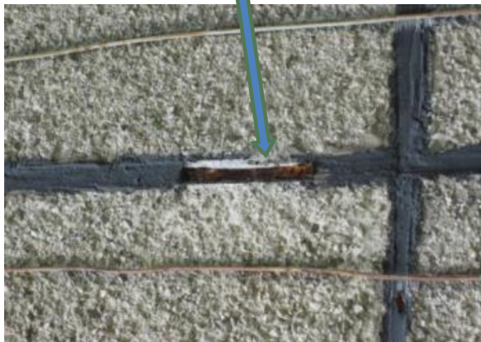
Crushed panel joints
